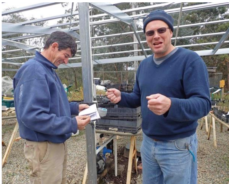
Kelvin and Jason work out how the installed system functions.
