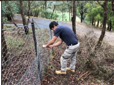
Kelvin also attaching the new mesh. TAG photos Don Vincent
