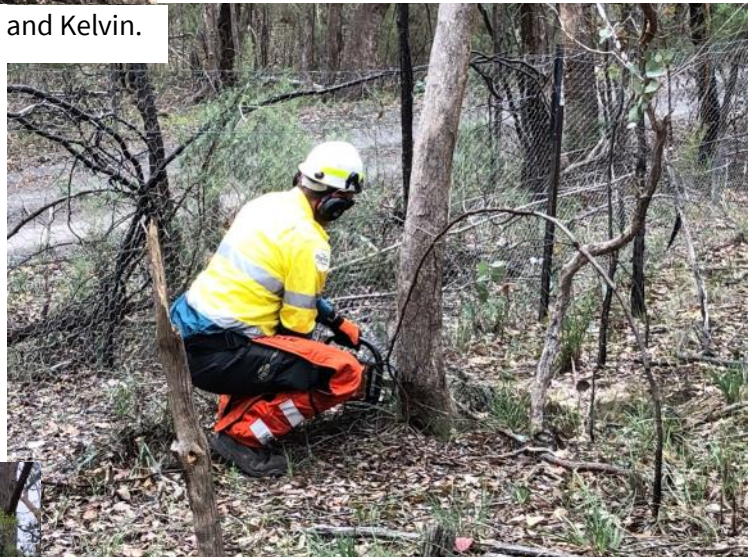
Parks Vic fire crew member
