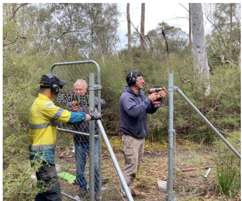
Phil, Brian and Kelvin working on the gate.
