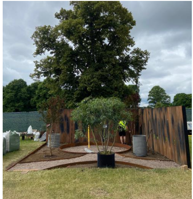
Above: the site in preparation
